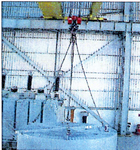
Picture 5 – Lifting of reactor by lifting lugs located on the crossarms.
